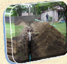
Residential Sewer Line Replacement
