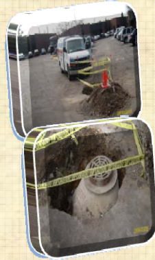
Commercial Man Hole Replacement
